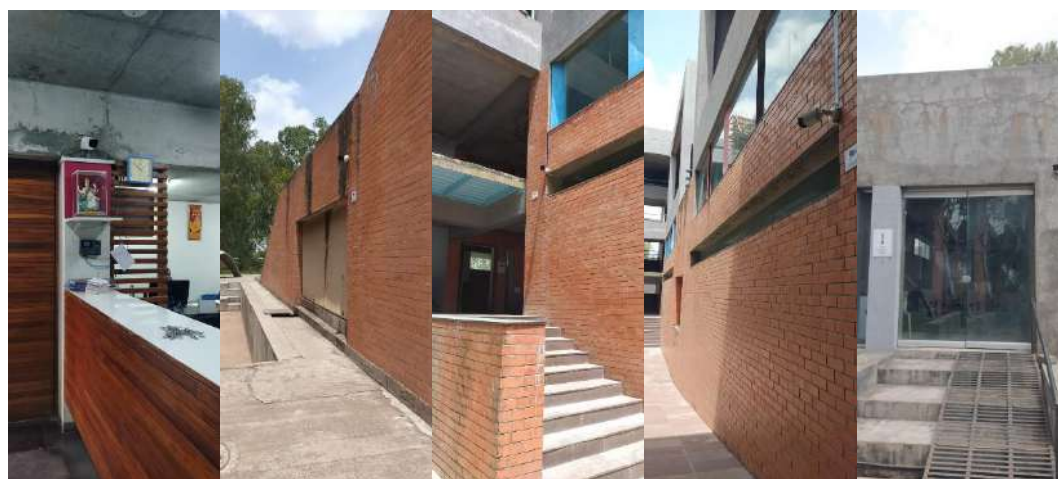
Installation of CCTV cameras in the campus
