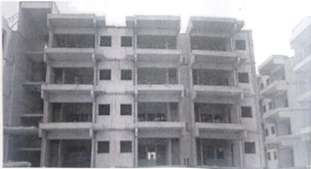
Fig.4: Mid rise precast paneled scheme at Bangalore (Source: NBM Media Publication, 2015)
