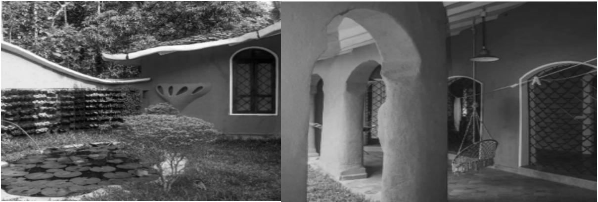
Image 2: Bodhi house Designed by Ar. Eugene Pandala made by the cob method of mud construction (Source: @eugenepandala)
