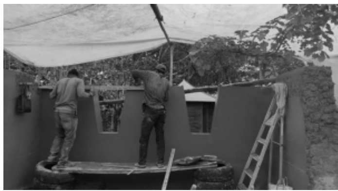
Image 1 : Ongoing project with experimentation of tessellations using cob in Pune, India. (Source : Studio Roots and Basics)
